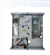
EXcel2 - 2 Reader, 1 or 2 Door Controller with 4A PSU
